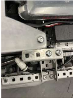
Steps 2 and 3: Intake attached to new screw joint
